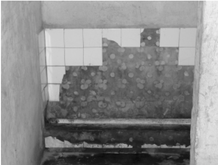
There are no functional toilet facilities at AllPay's Southwell pay-point
