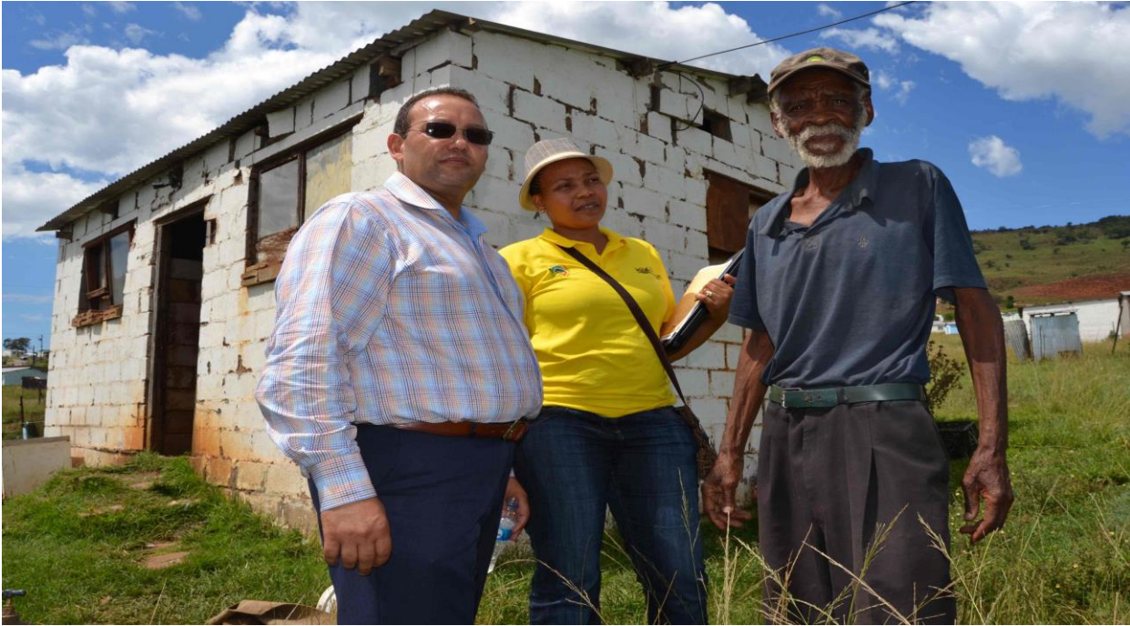
shoddy construction. Image source: daily Dispatch, March 2015
