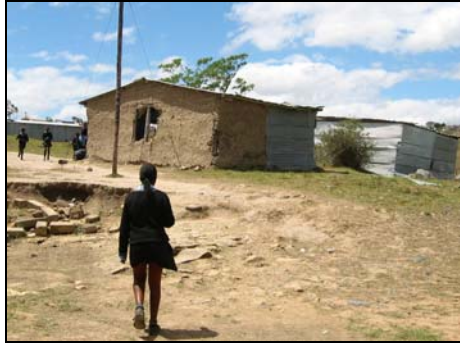
Mud and Zinc structured classrooms, Maganise JSS
