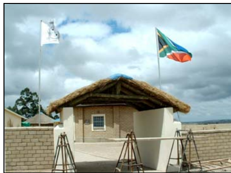
Incomplete, Bantwanana JSS
